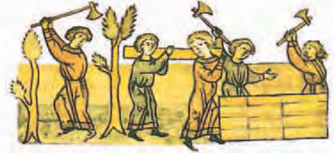
THE WALLS GO UP
